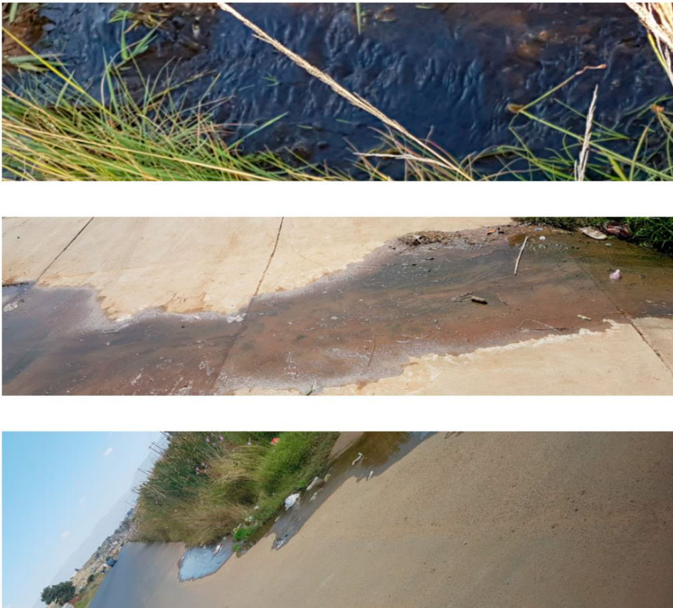
Figure 2. Water leakage flowing down the streets of Namahadi area in QwaQwa, South Africa (Source: authors).
