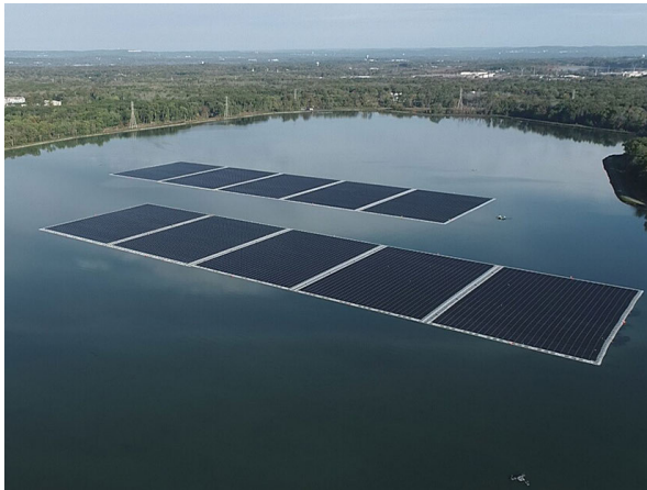
FIGURE 2. The largest FPV project in North America, in Canoe Brook Reservoir, with a total of 8.9 MW. Image credit: NJR Clean Energy Ventures.
